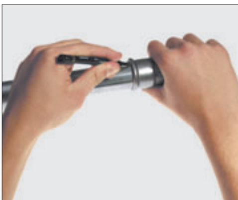
■ Marking insertion depth.
