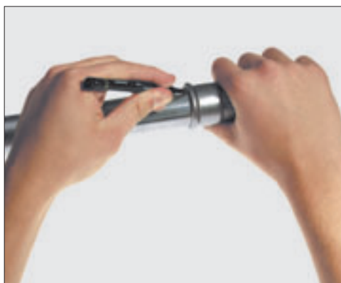
■ Marking insertion depth.
